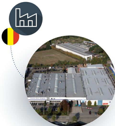
Structural production site Herentals, Belgium
